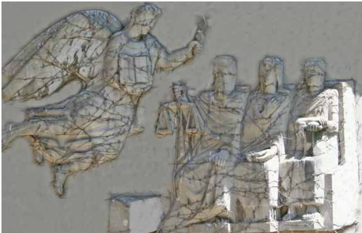
125-01 Queens Boulevard, Facade
