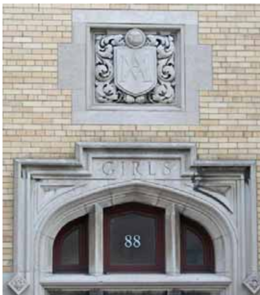
88-94 Visitation Place, Facade
